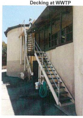
This project was initiated in FY 2014/15 but has been carried over to FY 2015/16 for completion. The scope of this project includes design and preparation of plans and specifications for the demolition and replacement of the decking and stairwell landing outside of the second story office space at the treatment plant. The design plans specifications have completed. Staff will be soliciting bids for the project soon and anticipates the project will be completed in the first quarter of FY 2015/16.
