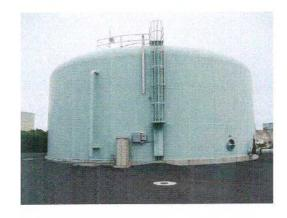
This budget item provides for water storage system improvements to District Water Tank No. 1. The proposed improvements include the installation of an internal tank mixer to reduce thermal stratification of stored water and eliminate short circuiting of fresh water from the supply inlet to the discharge outlet, allowing for proper mixing of new and aged water.
