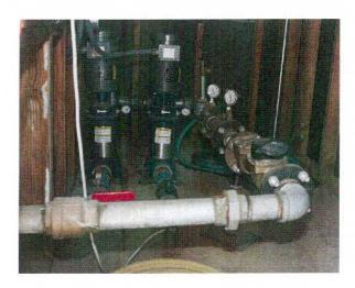
The existing booster pumps at the Lopez supply connection are marginally sized for existing maximum day demand requirements.
