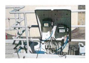
The scope of this project includes replacing the chlorine analyzer and chlorine dosing system. The new system will be monitored and alarmed through the Plant SCADA system and will offer redundancy should one of the components malfunction or fail.
