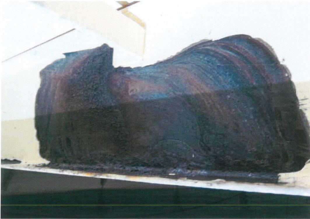
Typical view of roof support rafter on tank interior where coatings were removed with a scraper.
