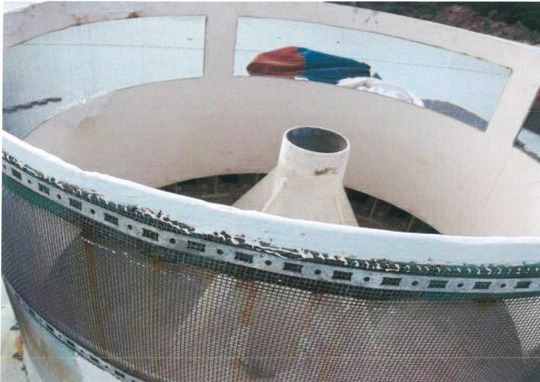
Top rim of the vent after application of epoxy. The screen was not removed because the existing clamp is corroded to the extent that it would have failed during removal.
