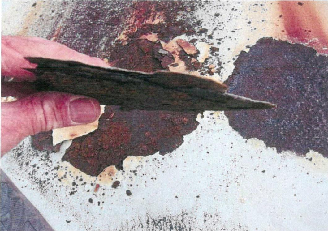
Typical corrosion location on exterior roof. Approximately 25 locations were repaired on the exterior roof.
