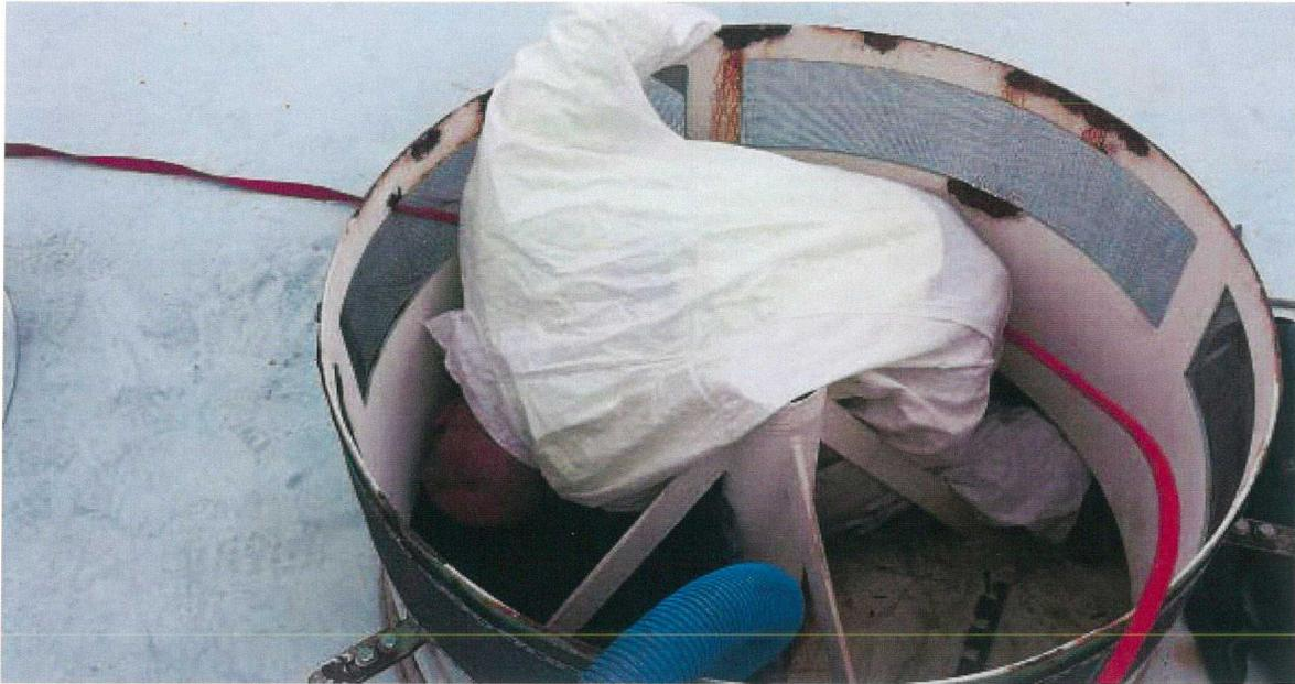
Corrosion removal in process on rafters inside of roof vent.
