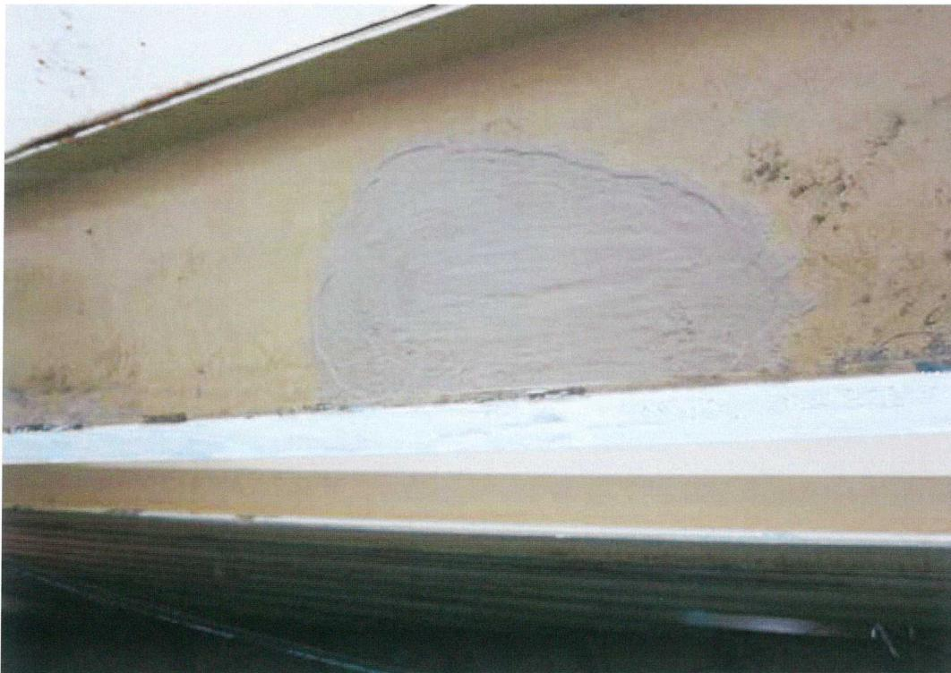
Typical spot repair on roof support rafter on tank interior. Approximately 100 similar locations were repaired.
