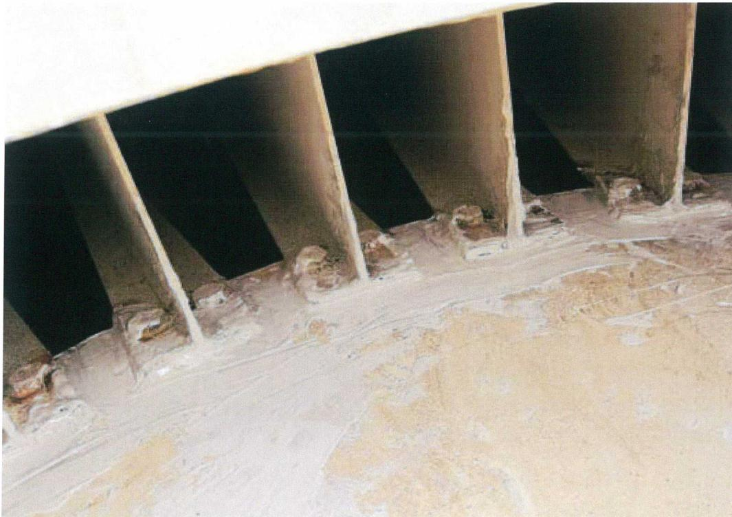
This is a typical view showing rafter ends after removal of corrosion and application of 100% solids epoxy. All rafters were spot coated in this manner.
