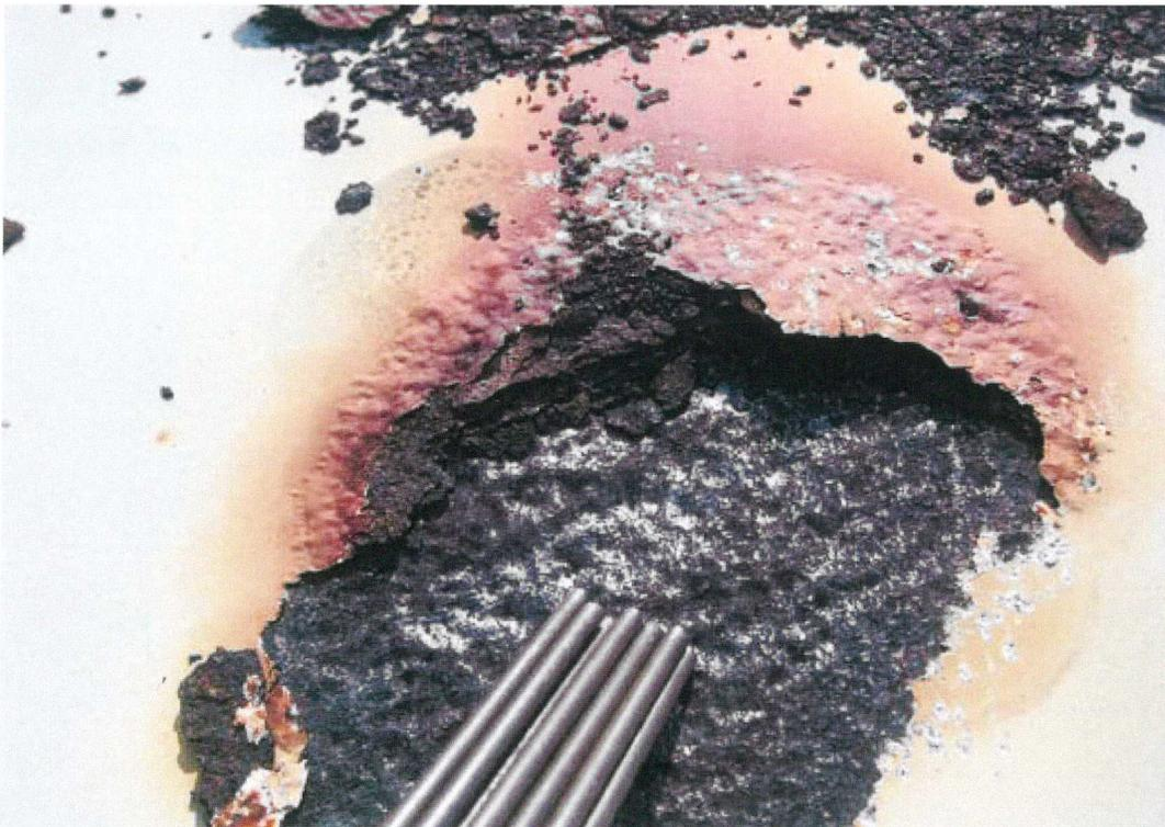
Preparation in process showing the amount of corrosion damage.
