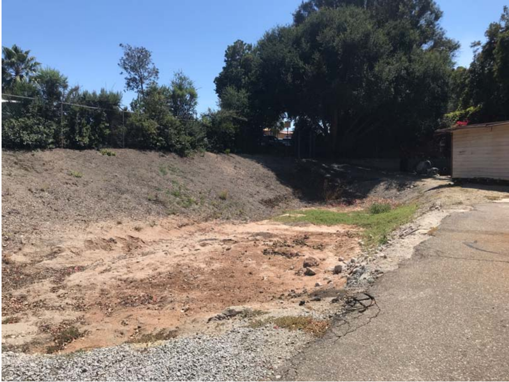
Photo 7. The project also involves installing a Side Stream Organic Loading Redundancy Treatment System in this location within the existing Wastewater Treatment Facility.
