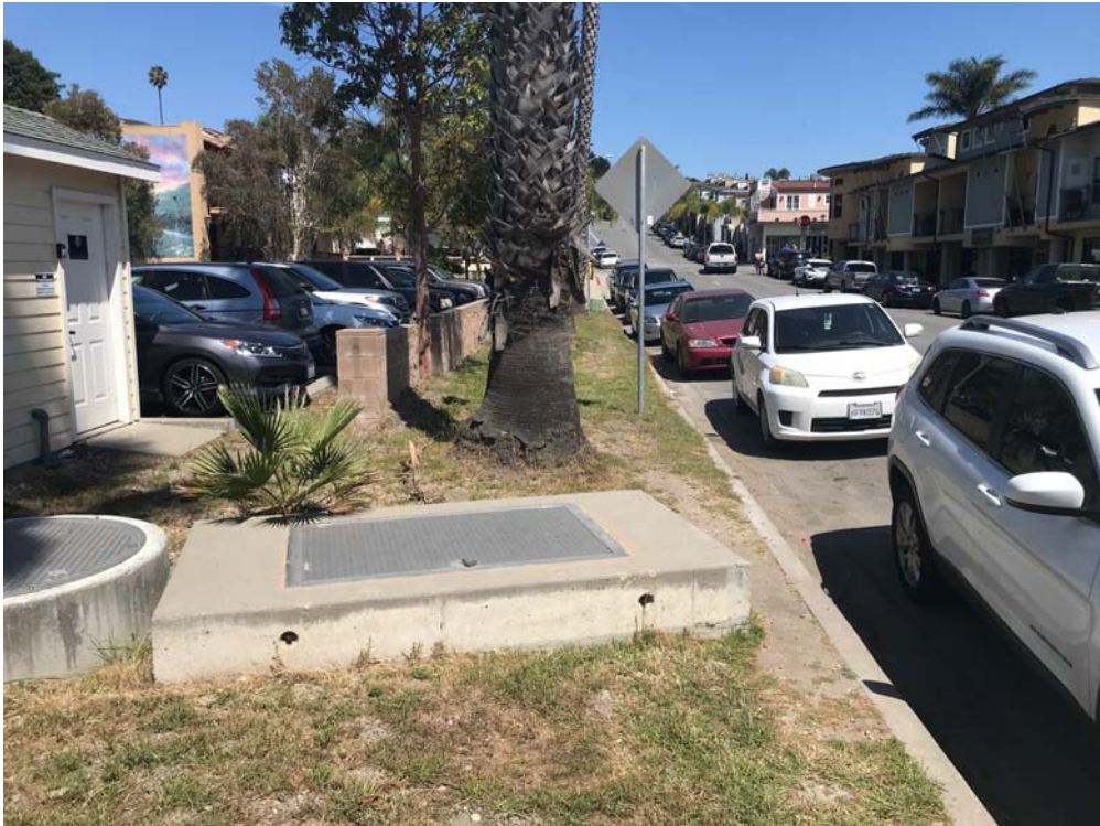
Photo 7. The FMRP would connect with existing infrastructure at this lift station on 1 st Street.
