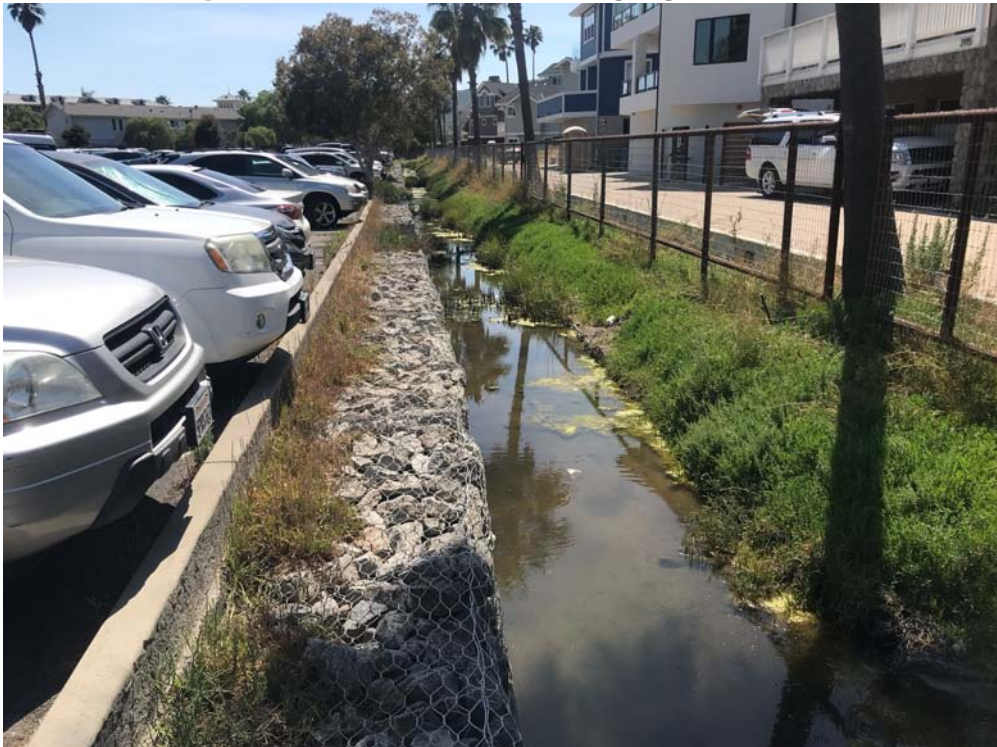
Photo 4. Southwesterly view of ditch where it transitions from concrete to earthen bottom and the new force main sewer line (FMRP) would be cross underground. Rock gabion baskets line both banks and salt marsh vegetation covered the northwestern (right) bank.
