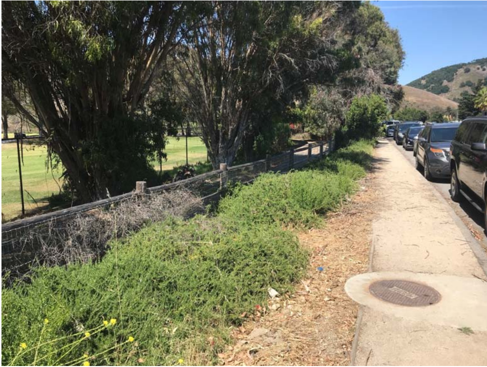
Photo 1. The Project would tie the new force main sewer line into an existing sewer line on Avila Beach Drive. Note landscaping and planted eucalyptus trees to the left.
