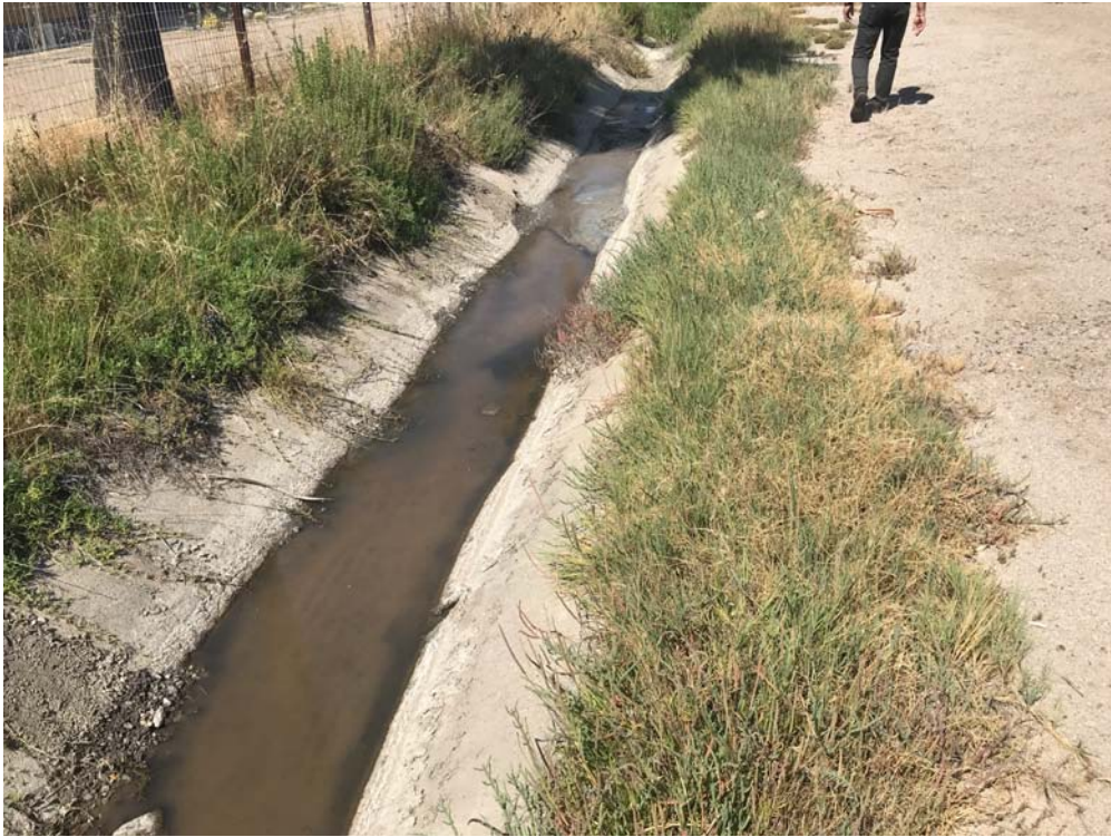
Photo 3. The stormwater ditch between Beach Colony Lane and Avila Public Parking Lot where it exists as a trapezoidal concrete channel lacking vegetation.
