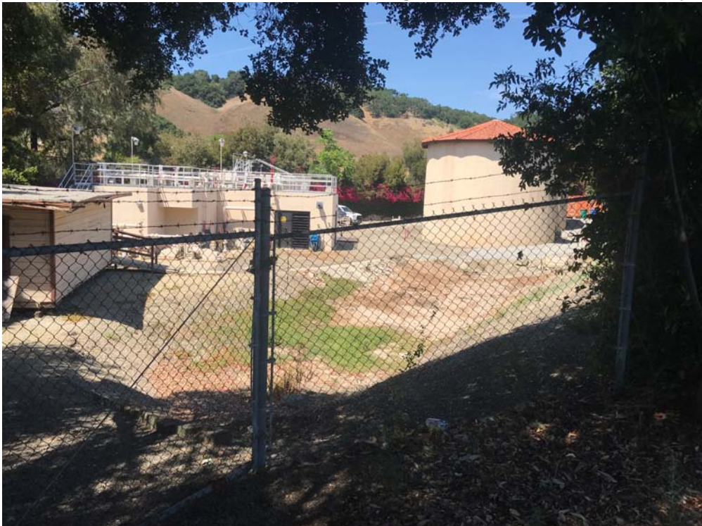
Photo 8. Additional view of the disturbance area for work within the existing Wastewater Treatment Facility. All construction activities would be sited in disturbed/developed areas and surrounding vegetation would be avoided.
